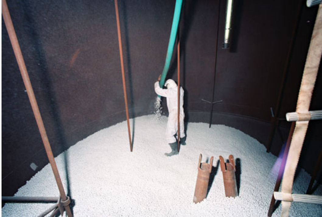
Loading the Fixed Bed MTG Reactor
